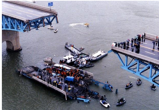
Collapse of the Seongsu bridge due to the welding failure (1994)
