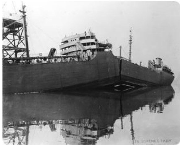
Brittle fracture on 1250 Liberty ships initiated at welds (50th)
